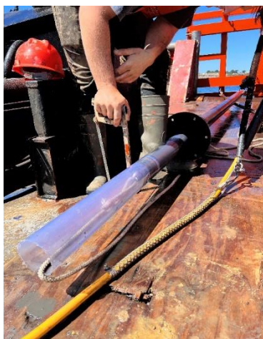
PVC pipe containing sediment pulled from the steel pipe
